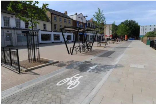
Image: Cycle lane in Lower Bridge Street.
